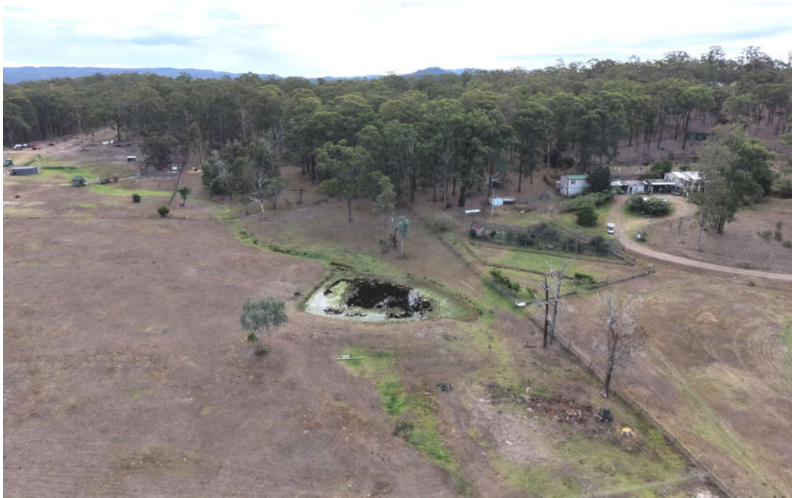
PHOTO 1 - SITE PHOTO LOOKING NORTHWEST
